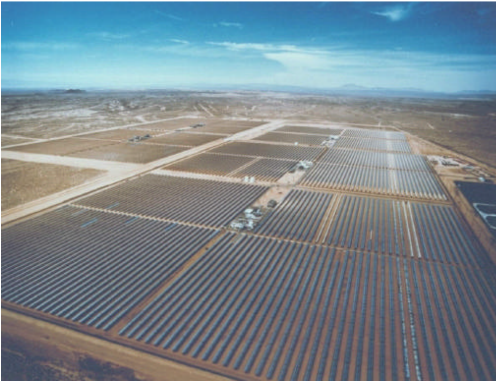
Figure 5: Aerial view of the solar thermal power plants at Kramer Junction in the US-Californian Mojave desert (photograph: KJC)
