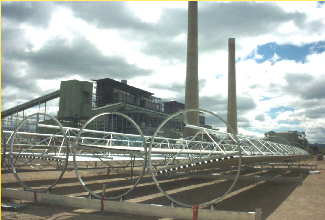
September 2003 : First installed reflector rows
