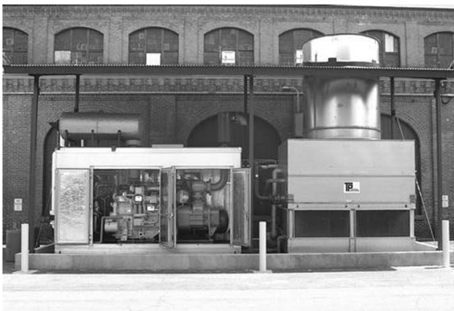
Since this natural-gas -engine-driven air compressor at the Watervliet Arsenal replaced the electric-motor driven units, significant energy savings have been realized.
